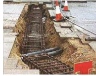
VSB foundations around underground services CPNI 2010
