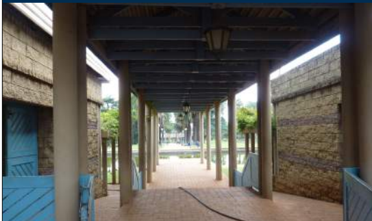
Are the opportunities for offenders to utilise access and escape routes limited? Is the level of ease with which potential victims could find escape routes enhanced?
