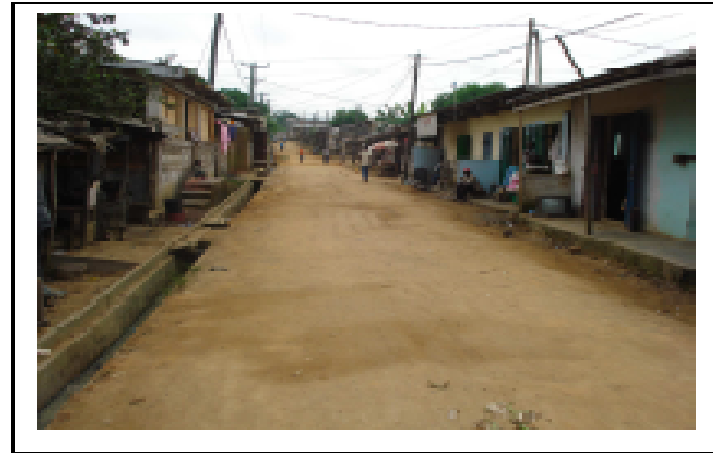
Roads constructed (December2008)
