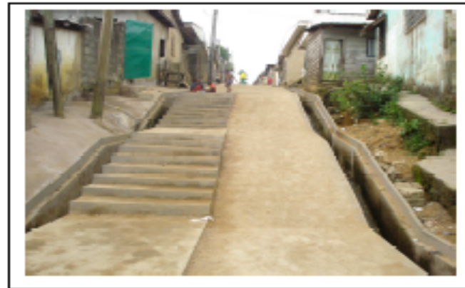
Upgraded road (December2008)
