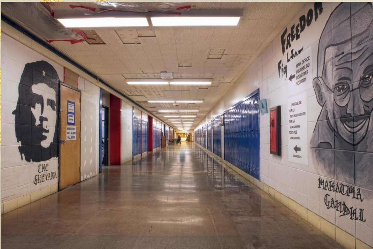
Hallway prior to modernization (Photo copyright reference for this attached image below: Rene Berndt, Mahlum)
