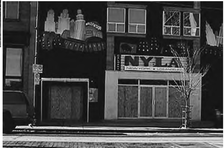
Figure 4 Boarded up exterior windows, 2003
